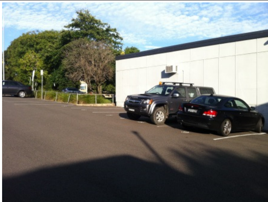
Photo 5.1.6 – Portion of asphalt car park, facing north west
