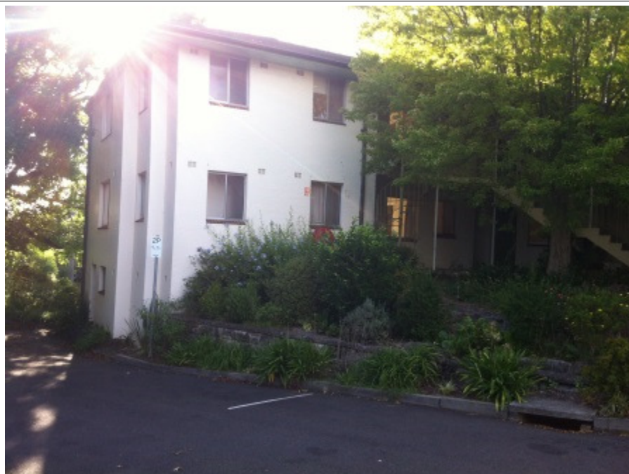
Photo 5.1.3 – Double storey residential apartment building, northern side
